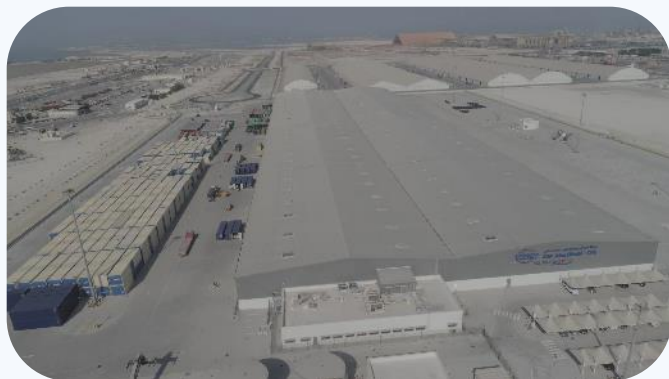
CSP Abu Dhabi CFS Phase 1
