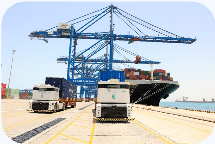
CSP Abu Dhabi Terminal
