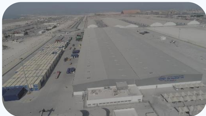
CSP Abu Dhabi CFS Phase 1
